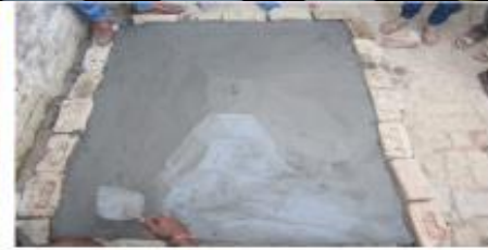
Fabrication of a Ferro-cement Roof top for a Toilet under transfer of technology by Anar Devi Khandelwal Mahila Polytechnic, Mathura at village Chaumuha, Chhatikara near Vrindavan
