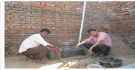
Construction of a smokeless chullah under transfer of technology by Anar Devi Khandelwal Mahila Polytechnic, Mathura at village Chaumuha, Chhatikara near Vrindavan
