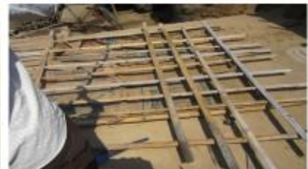
Fabrication of low cost roof using local materials like bamboo and gunny bags
