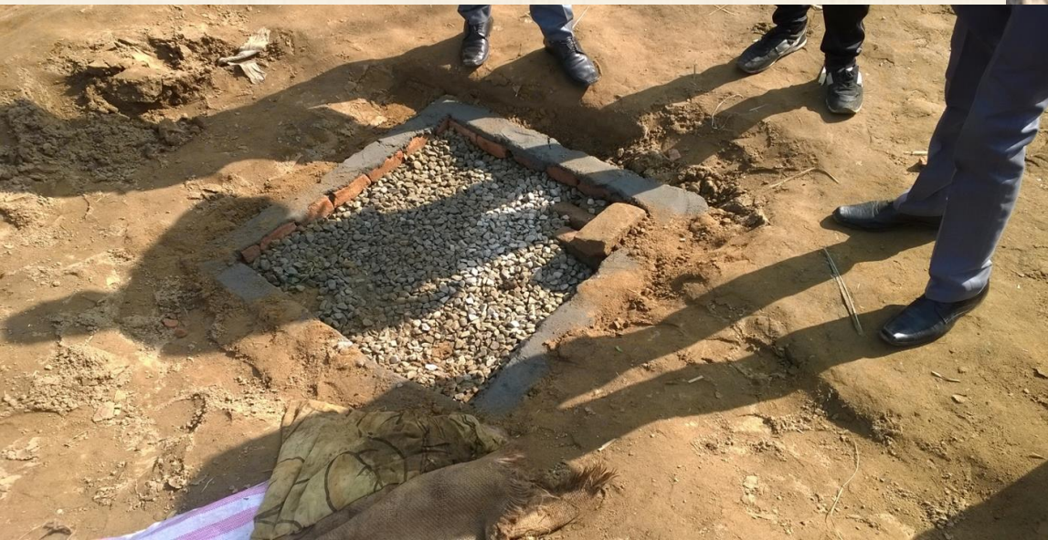
Wastewater Disposal System: Village Chaukpuri, UP
