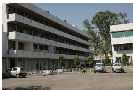
Three Storeyed Hostel Block
